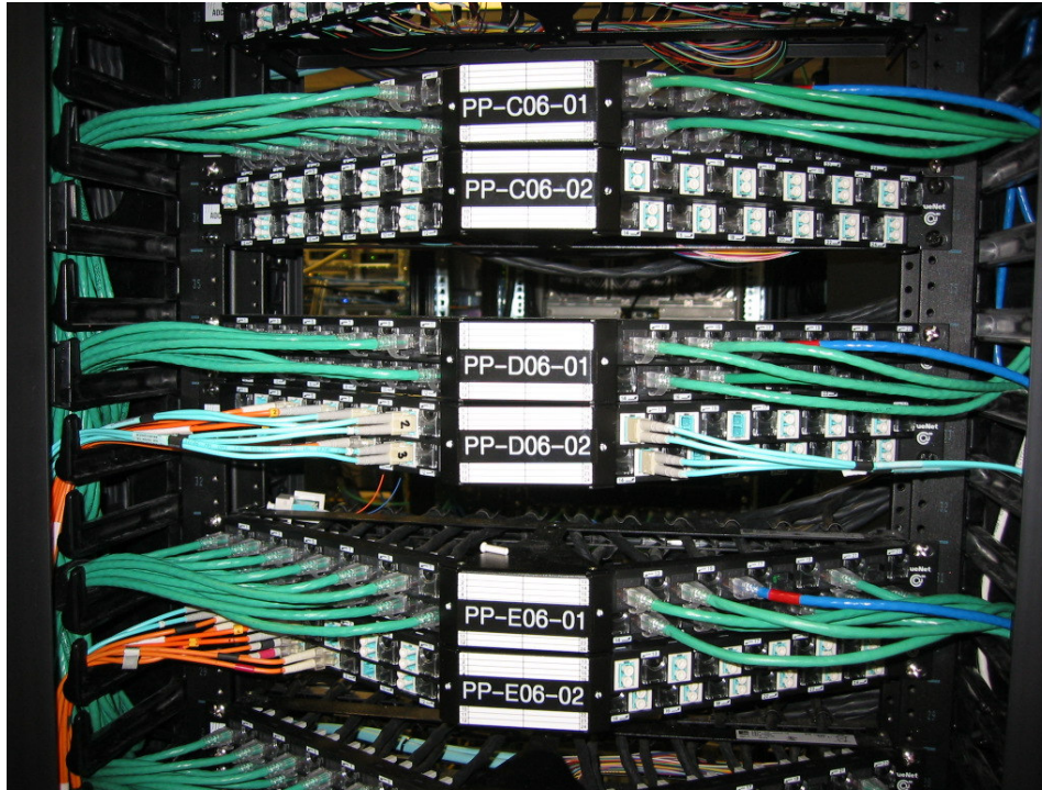
Figure 6. Angled patch panels allow cables to be routed directly into the vertical cable managers.
