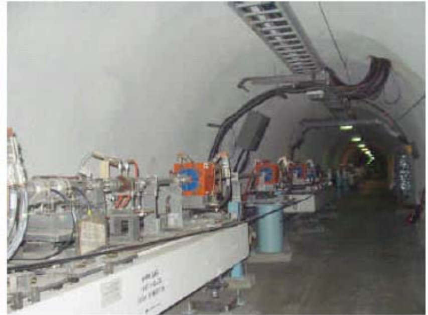
Instrument Section, looking upstream.
