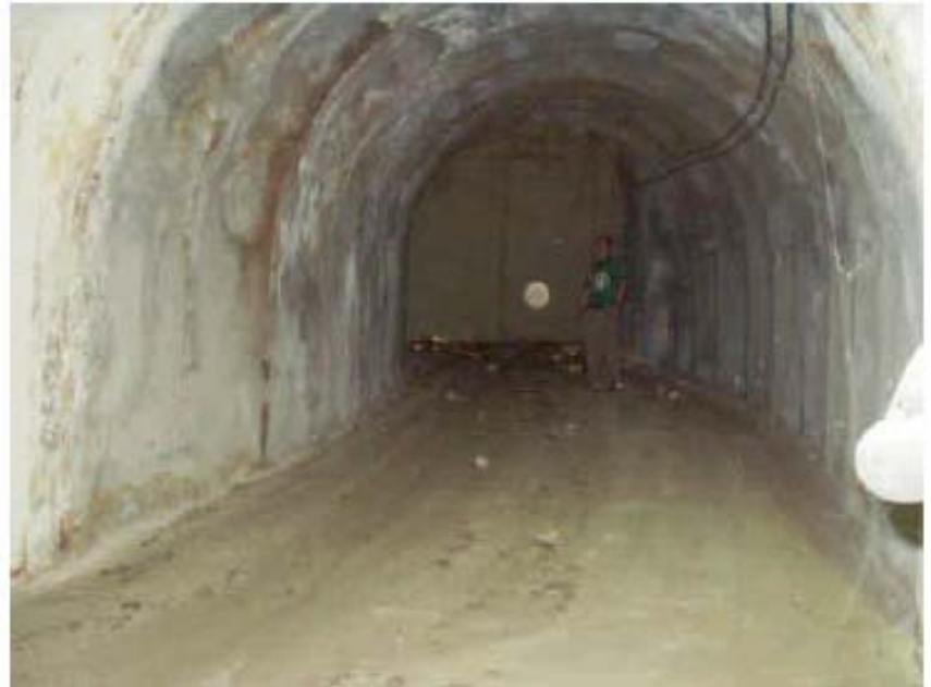
Southwest Adit tunnel, leading to removable shielding wall.
