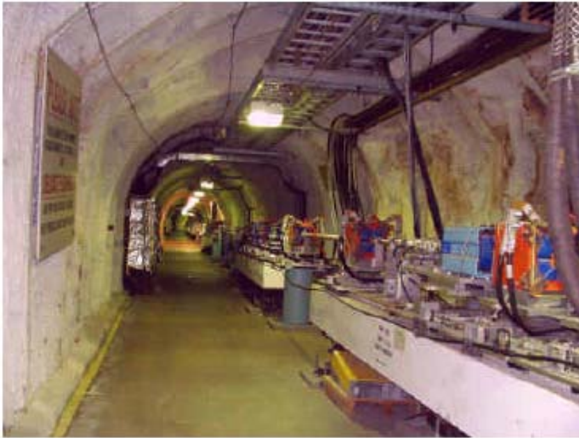
Instrument Section, looking downstream. Floor slopes slightly downward.
