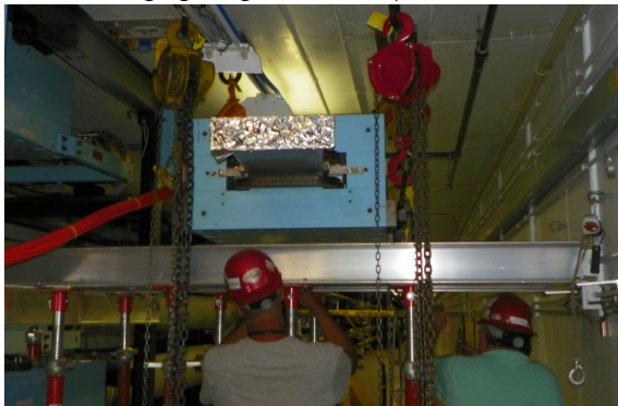
Dogleg magnet removal/insertion:
