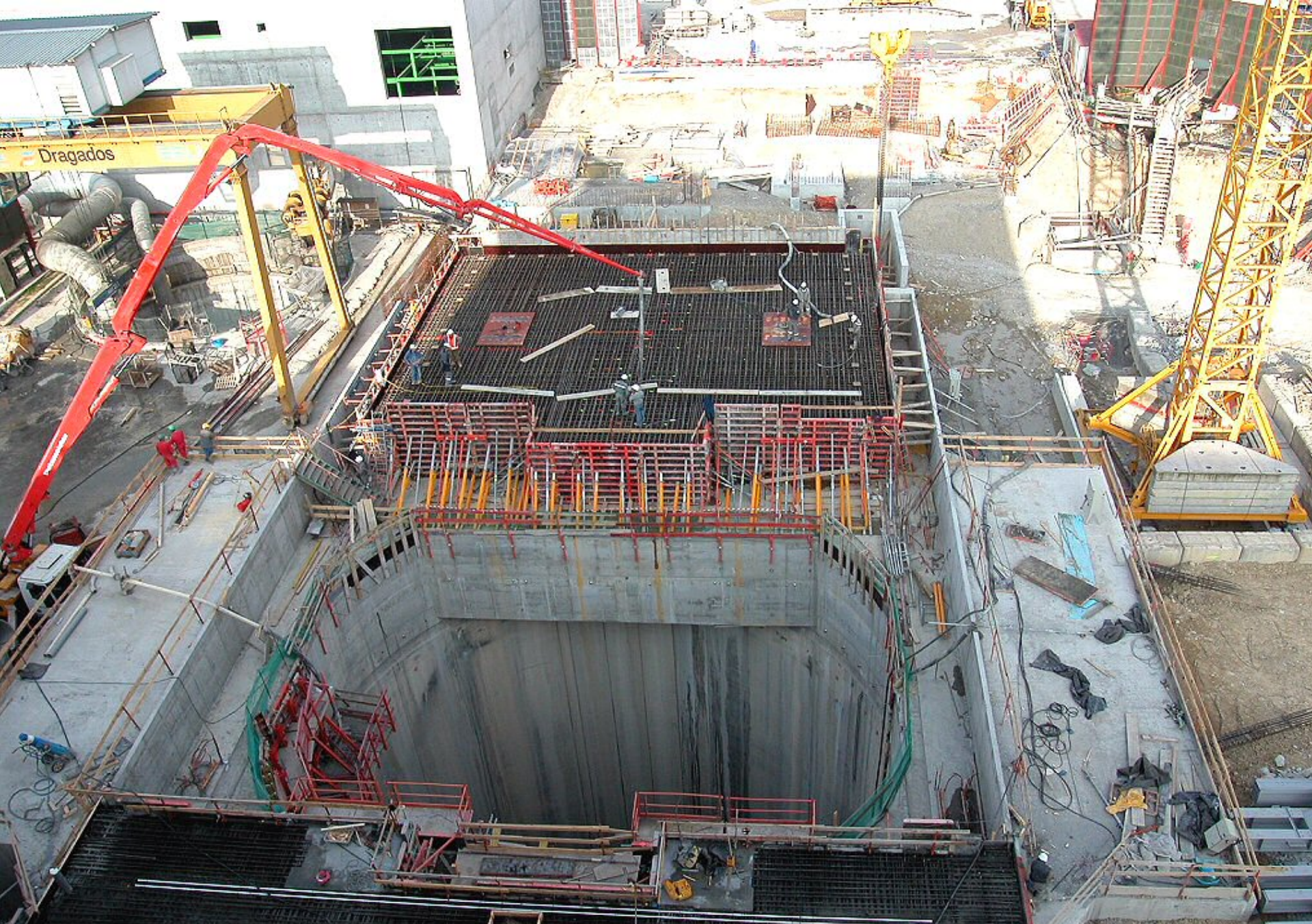
LHC Point 5 - Concreting of PX56 Bouchon - 30-03-2004 - CERN TS-CE
