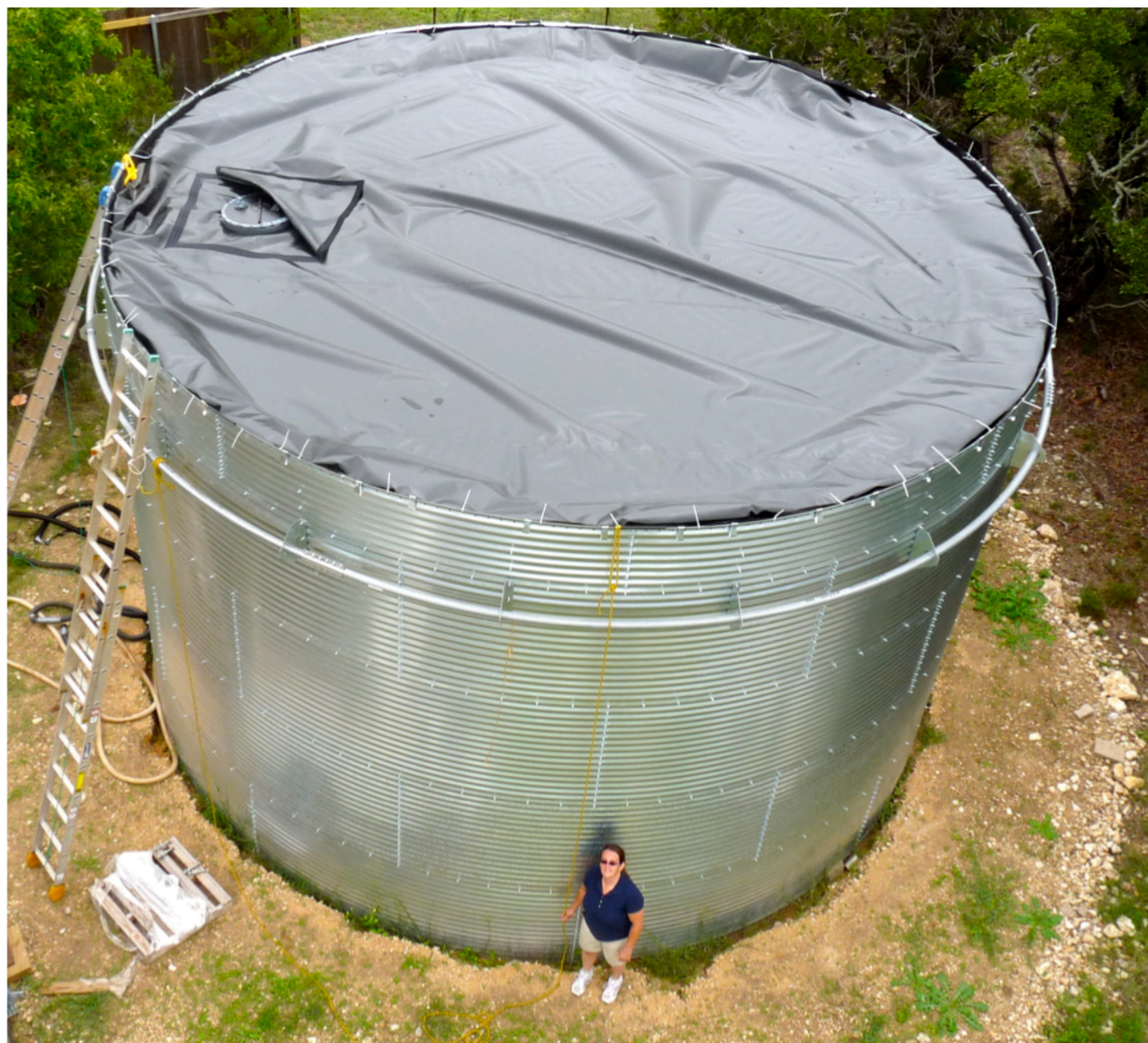
Figure 2: The first full size HAWC tank of 7.3m diameter with a custom designed bladder. Filled in Austin Texas with 200,000 liters of water and light leak tested with a HAWC PMT.
