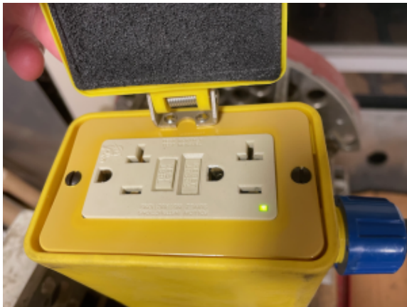
Fig 1: 110V ceiling breaker and dropdown cable to the yellow quad distributed outlets. Ceiling breaker limit can often be read from the switch knob on it, typically 20A. Each of the quad outlets is also 20A compliant as indicated by the T-shaped leg. Each outlet can be considered to be equivalent to a wall socket.
