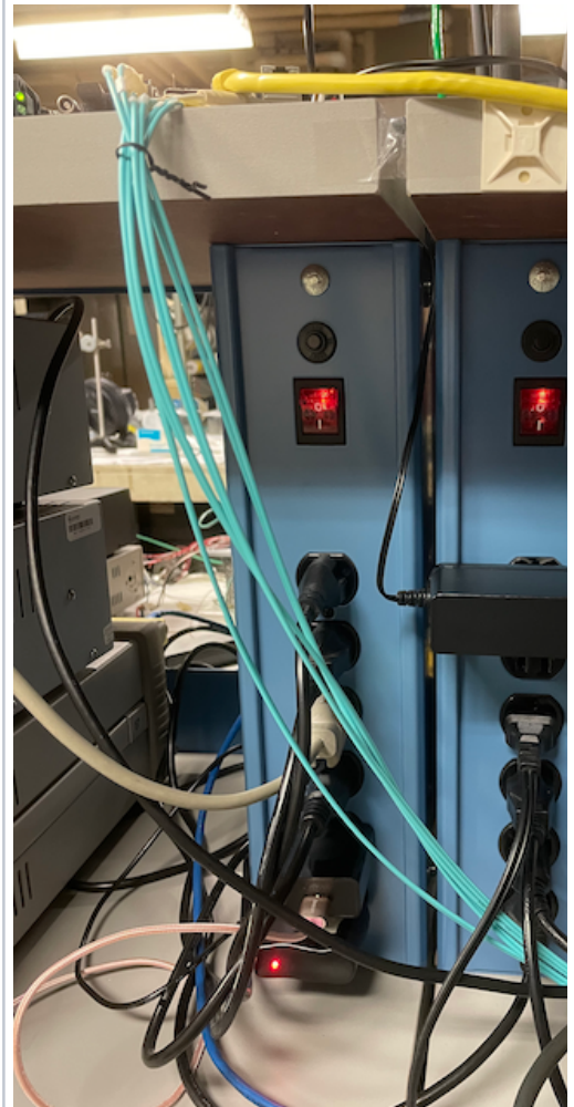
Fig. 2: The bench outlets are NOT equivalent to wall socket but power strip. They are collectively served by just one line at the the dropdown yellow box. DO NOT plug in any power strip or e. sockets. High power appliances (>~500W) should go to the yel directly.
