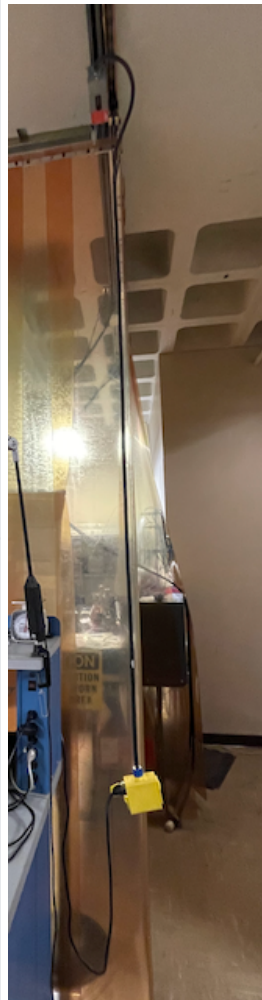
Fig 1: 110V ceiling breaker and dropdown cable to the yellow quad distributed outlets. Ceiling breaker limit can often be read from the switch knob on it, typically 20A. Each of the quad outlets is also 20A compliant as indicated by the T-shaped leg. Each outlet can be considered to be equivalent to a wall socket.
